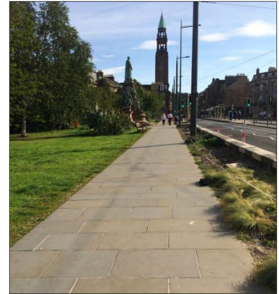
Paving Improvements and Restored Walls at Coates Gardens, West End Princes Street.
