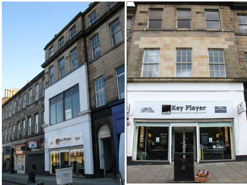
13 Elm Row Shop Front Restoration
