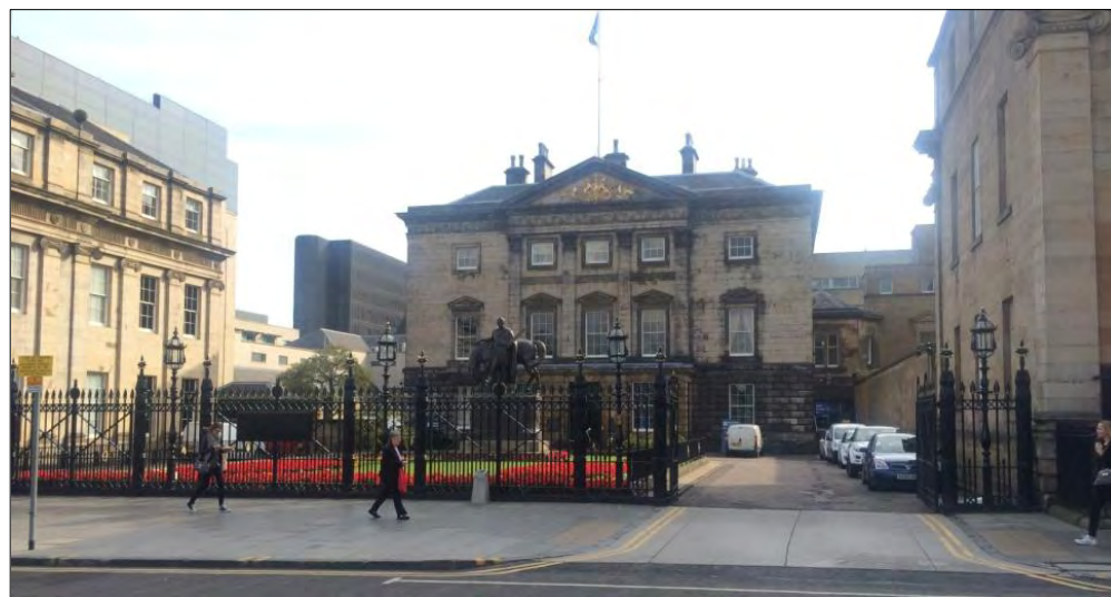
Royal Bank of Scotland Building, St Andrew Square
